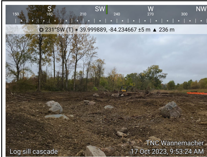
Photograph 1: Log sill cascade construction near Sta 13+50.
