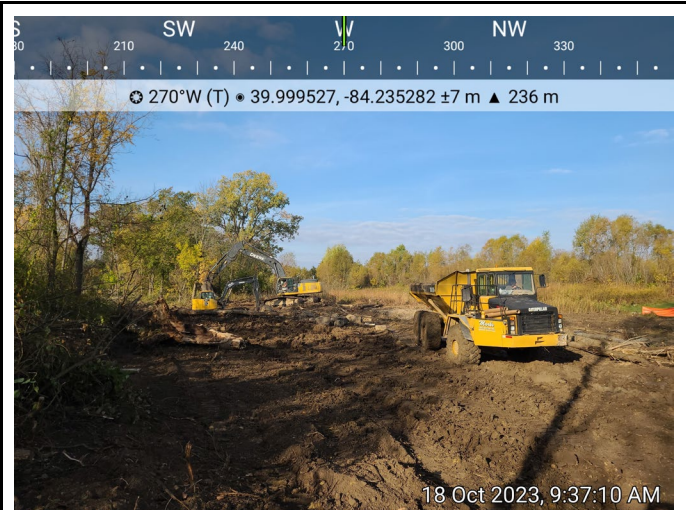
Photograph 2: Rough grading the new channel alignment upstream of Sta 12+00.
