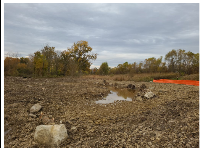
Photograph 4: Looking upstream at toewood revetment with root wads, across from finished floodplain.
