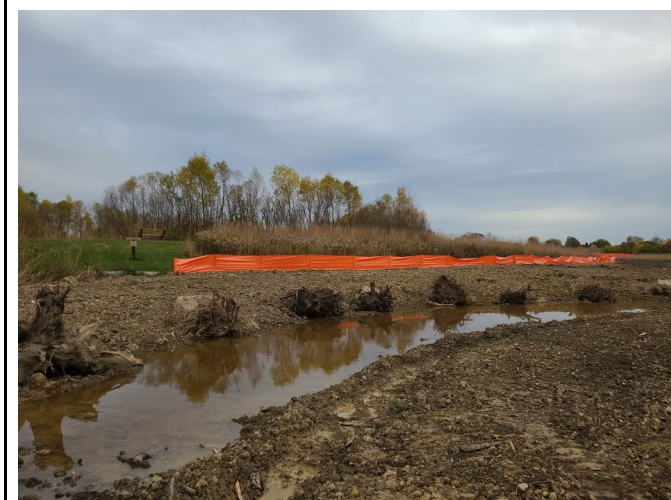
Photograph 3: Toewood revetment installation near Sta 16+00.
