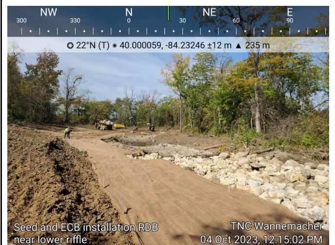
Photograph 4: Seed and blanket installation along the bankfull floodplain, right descending bank.
