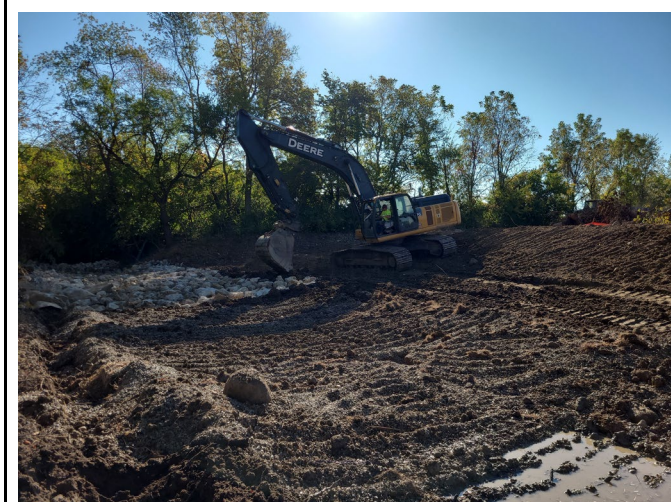
Photograph 3: Installing "reinforced bed mixture" at runs and glides near Sta 23+50.
