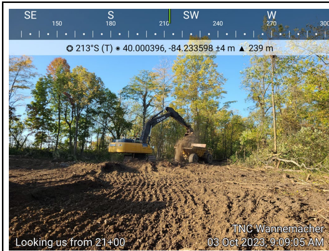
Photograph 1: Construction of the new channel from Sta 20+00 to 18+00.
