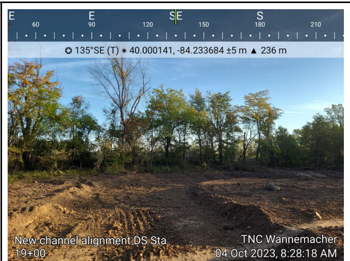
Photograph 2: Rough grading new channel alignment downstream from Sta 19+00.
