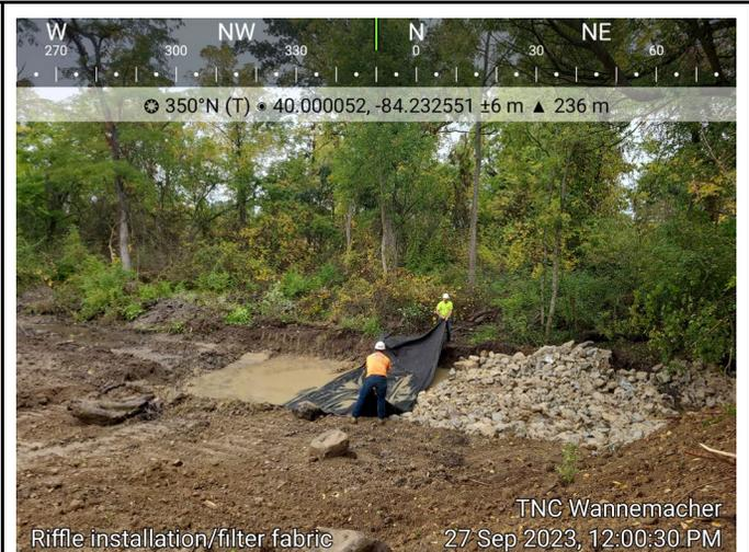
**Photograph 6:** Installation of filter fabric under lowermost Newbury riffle, near Sta 24+00.
