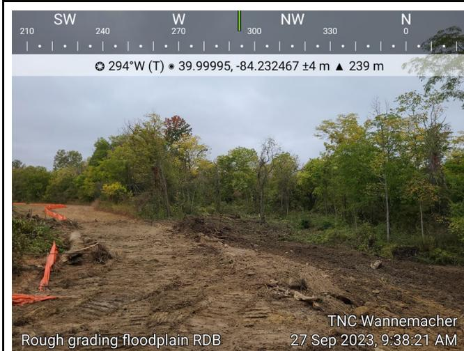
**Photograph 3:** Rough grading of bankfull bench along RDB near Sta 23+00.
