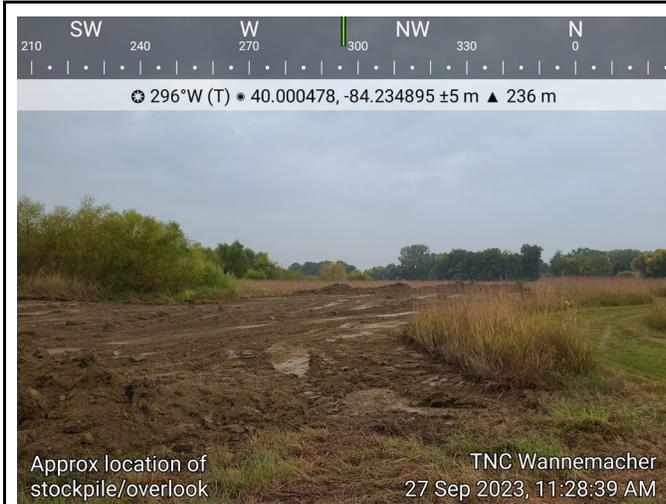
**Photograph 5:** Clearing and preparation of subgrade for soil stockpile/central overlook area.
